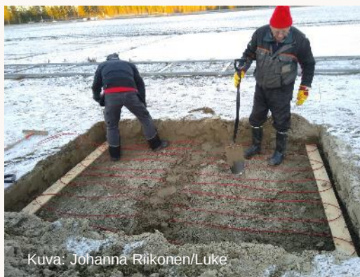
Installing soil resistance cables
