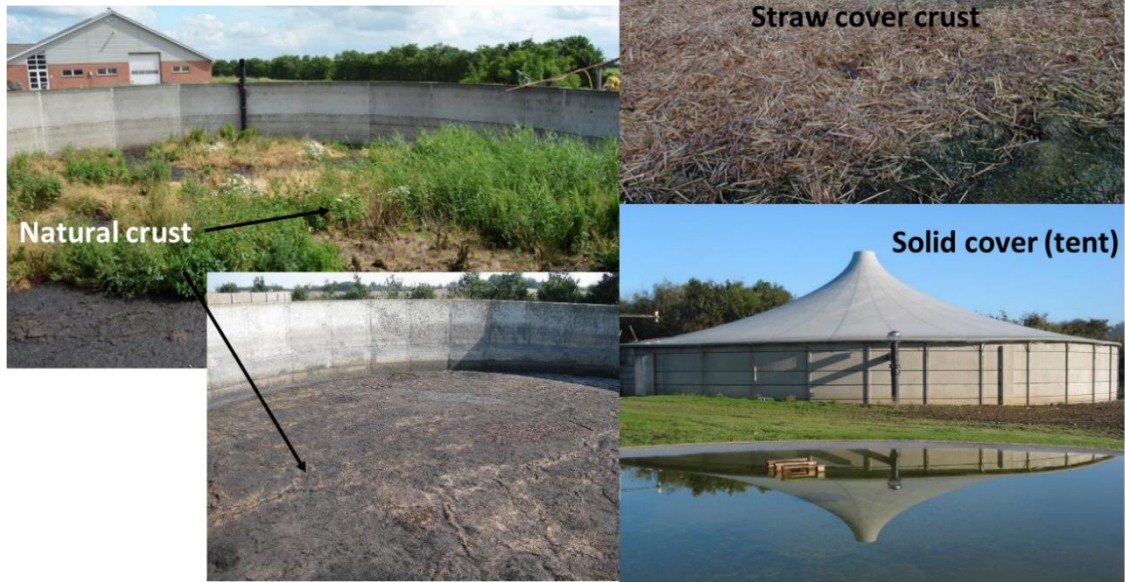
Figure 3.1. Examples of cover of slurry tanks. Pictures: SEGES, Denmark.
